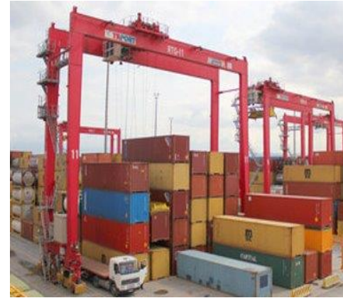
Rubber Tyred Gantry crane (RTG)
